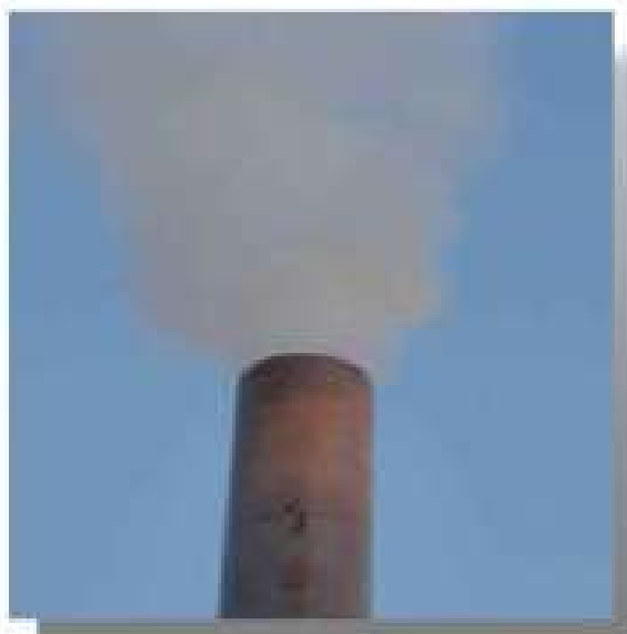
Before Running Gas Disposal System
