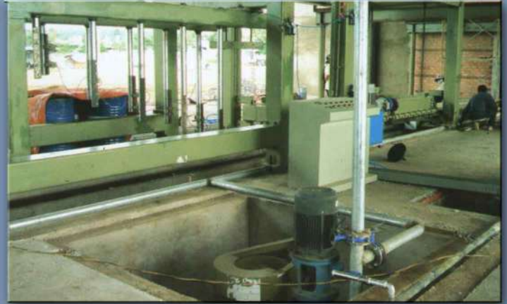
INSTALLING CUTTING MACHINE
